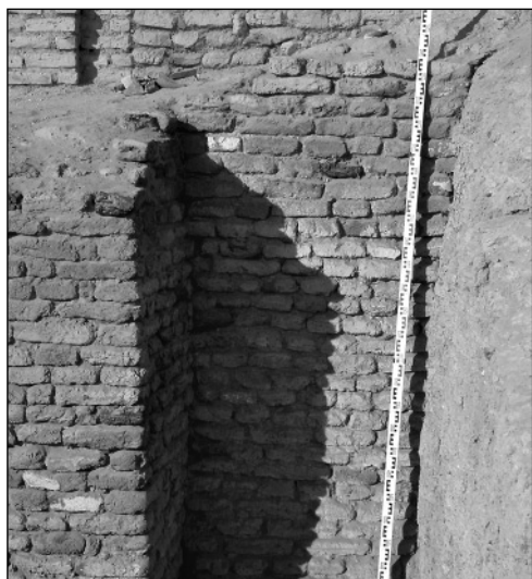
Fig. 4. Red-brick inner reinforcement of the monastery enclosure wall (Photo J. Świącicki)
