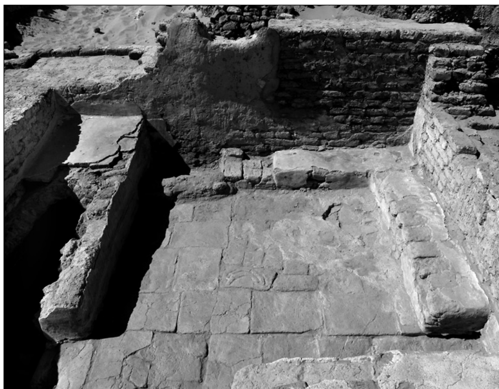
Fig. 3. Monastery Church, northwestern corner room, view to the west and longitudinal section through the room looking west (Photo D. Gazda; drawing M. Puzskarski, after original documentation by D. Gazda and A. Cedro )
