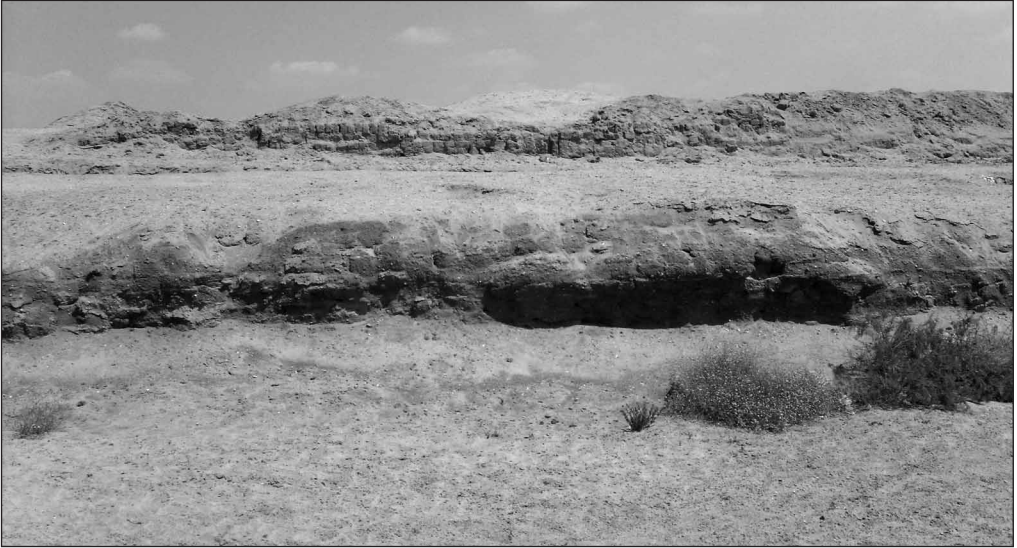
Fig. 2. Southern defense wall of the Ramesside fortress: Petrie's "wall 2" (in front) and "wall 3" (in the background) (Photo S. Rzepka)
