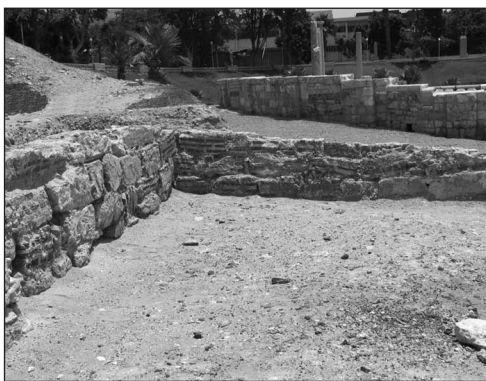
Fig. 5. Dump-retaining wall in central part of the site, view from the north (Photo G. Majcherek)
