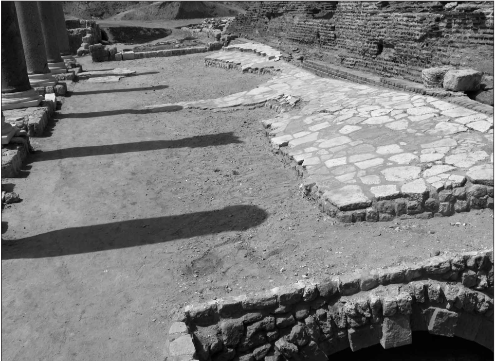
Fig. 14. South façade of the bath and adjoining passage, after conservation, view from the east (Photo G. Majcherek)
