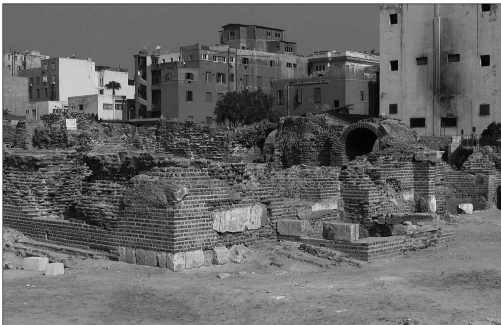
Fig. 12. East façade of the Late Roman Bath after conservation, view from the southeast (Photo G. Majcherek)
