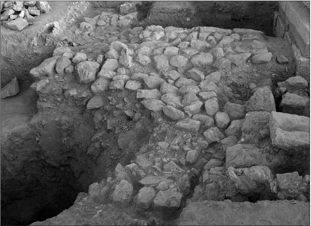
Fig. 3. Foundation of an earlier sacral structure in the northwestern corner of the cella (note mouth of cistern at bottom right) (Photo M. Gawlikowski)
