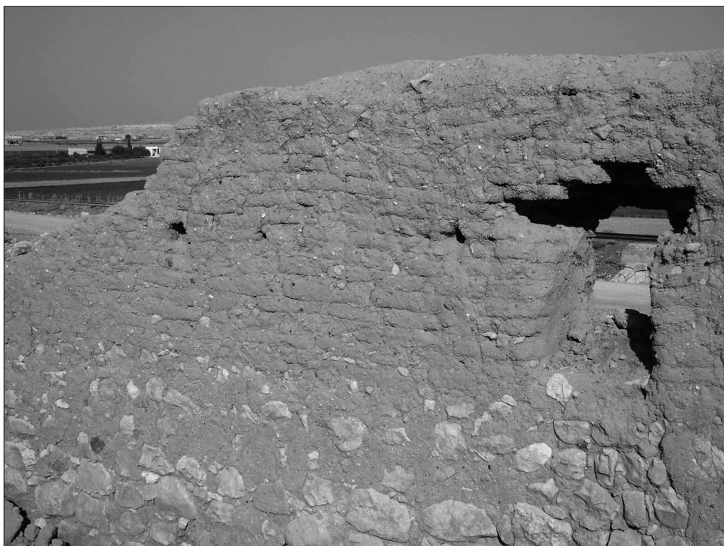
Fig. 7. Example of modern stone wall with superstructure made of mud bricks. Qaramel village (Photo M. Białowarczuk)
