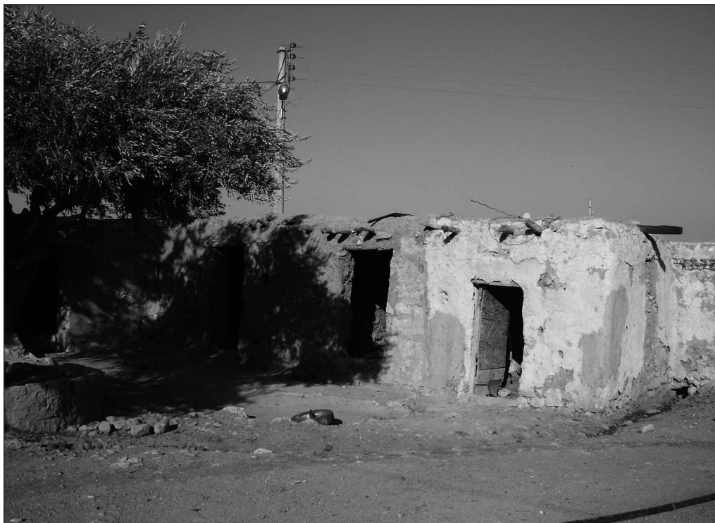
Fig. 3. Storage buildings made of pisé . Qaramel village (Photo M. Białowarczuk)
