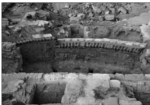
Fig. 3. Outer wall of the kiln, inboard face (left) with new mud-brick infill and brick and stone coping, and outboard face (right) with new retaining wall and coping (Photo Jack M. Kucy)
