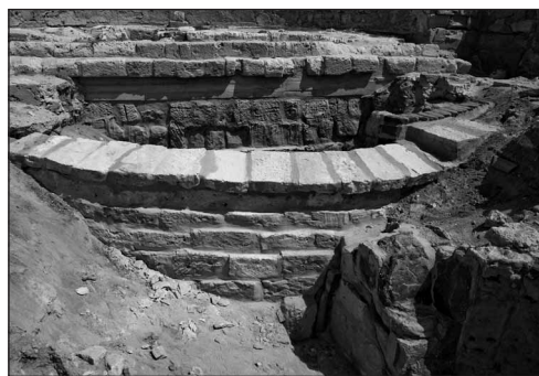
Fig. 3. Outer wall of the kiln, inboard face (left) with new mud-brick infill and brick and stone coping, and outboard face (right) with new retaining wall and coping (Photo Jack M. Kucy)
