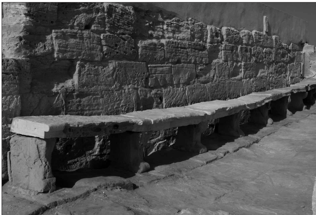
Fig. 8. Benches in the South Portico, state after full restoration in 2007 (Photo S. Medeksza)
