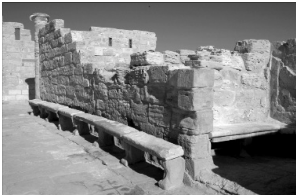
Fig. 8. South portico of the main town square with the back bench, after restoration in 2008 (Photo P. Zambrzycki)
