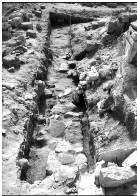
Fig. 3. Foundation of the northeastern corner of House 1 after clearing for conservation, view from the west (Photo P. Zambrzycki)
