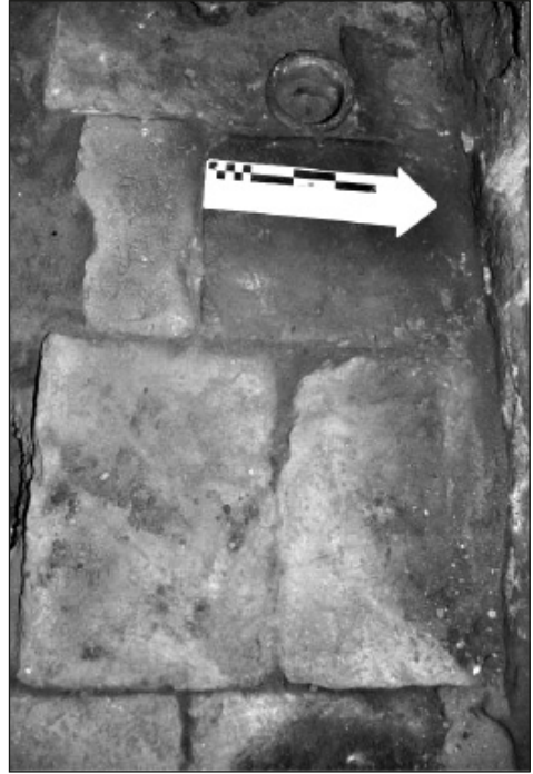
Fig. 1. Draining pipe in the ceramic pavement of the prothesis against the north wall, below a lamp niche (Photo B. Żurawski)
