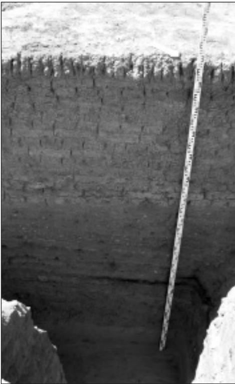
Fig. 3. Trench IX/2. Outer face of curtain wall (Wall II), view from the southeast
