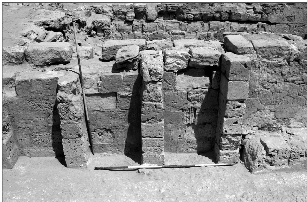
Fig. 2. North wall of the north aisle with presumed buttresses (Photo P. Suszek)
