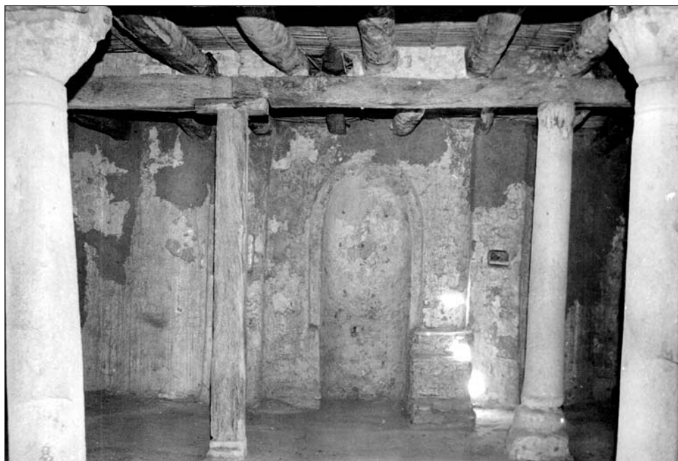
Fig. 13. Mosque: central room with mibrab on the first floor (Photo W. Jerke)
