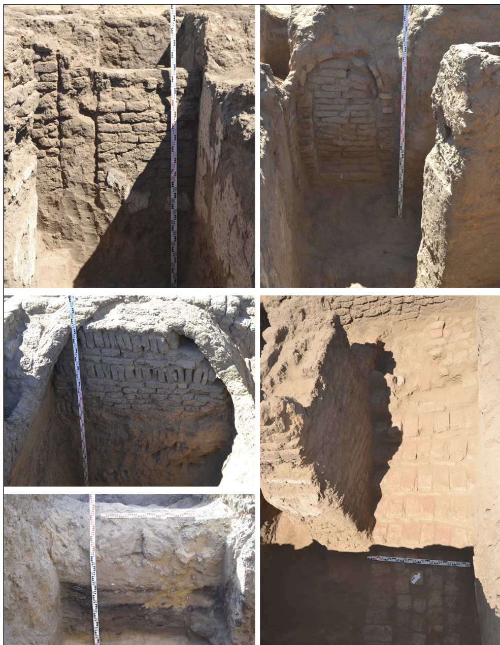
Fig. 3. House SW1: clockwise from top left, room 5, northeast wall including partition wall; room 4, door jamb on the west side; stairs in room 4; section of the fill in room 1; bricklaying course beneath the vault of room 3 (Photos E. Skowrońska, M. Drzewiecki)
