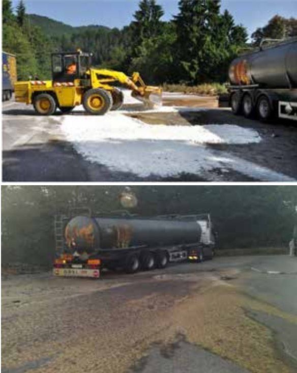
FIGURE 7 NEUTRALIZATION OF NITRIC ACID LEAK HYDRATED LIME
