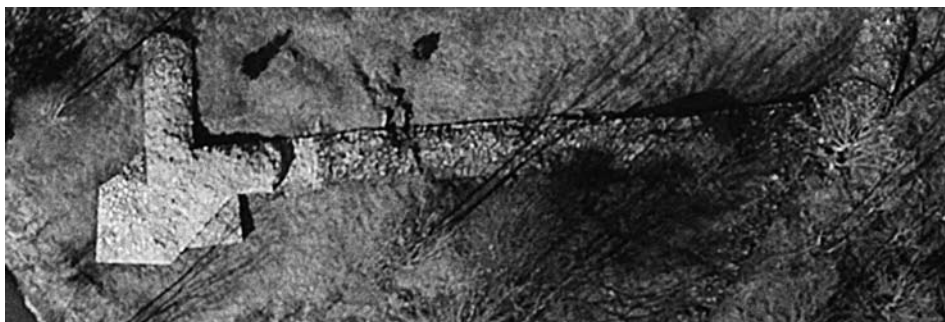
Fig. 20. The southwestern tower on the wall of the Ad Pirum fortress showing two chronological phases of its construction
