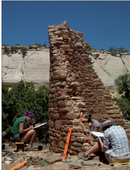
Figure 5. Tower at the Site 5MT181 (Mad Dog Tower) during the documentation by Sand Canyon-Castle Rock Community Archaeological Project in 2011. Photo by R. Palonka
