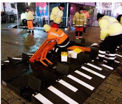
Image 8. Installation of temporary barriers as part of the security preparations for a public event, and a trial placement of barriers (Warsaw).
